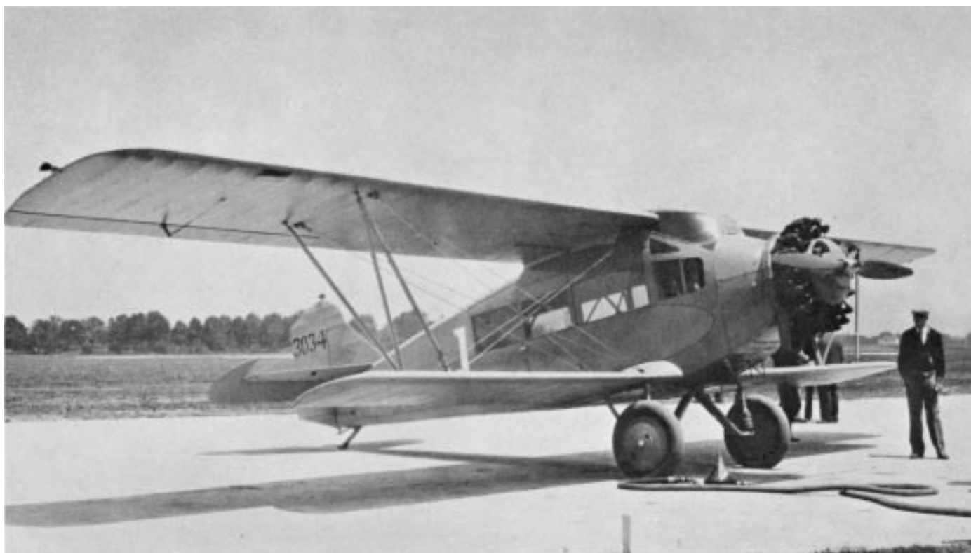
The Buhl Airsedan, Tour #1, Registration #3034. This "tail number" indicated the plane was identified and listed with the Department of Commerce, as required by the Air Commerce Act of 1926. "C" and "NC" license designations followed, as manufacturers proved their ships in airworthiness tests for an "Aircraft (or Approved) Type Certificate" which the Act required for use in interstate commerce.
